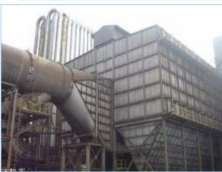
• Drop Out Box, Water-Cooled Duct, Fixed Duct
